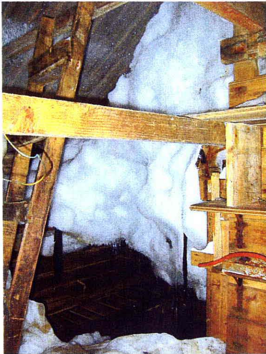
BEFORE – NOTE CAVAIITY UNDER ICE MASS
