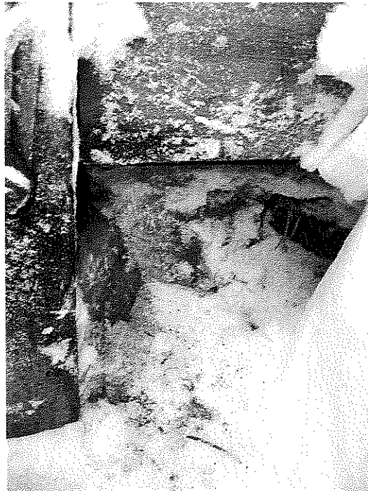
SOLID ICE UNDER FLOOR STRUCTURE
