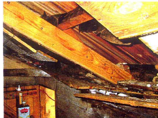
NEW SECTION STITCHED TO SIDE OF BROKEN RAFTER
