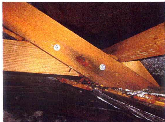
FIXING OF NEW TIE TO RAFTER
