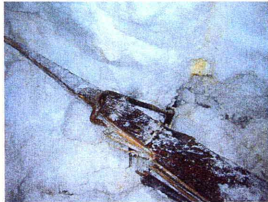
FRACTURED CONNECTION AT LOCATION OF COLLAR TIE JUNCTION
