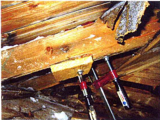
SECTIONS OF RAFTER RECOVERED AND ORIGINAL LOCATIONS DETERMINED
