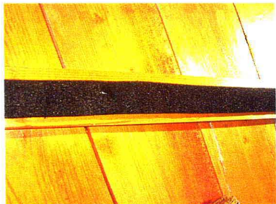
DETAIL OF COVER BATTEN AND FOAM STRIP BEFORE FIXING
