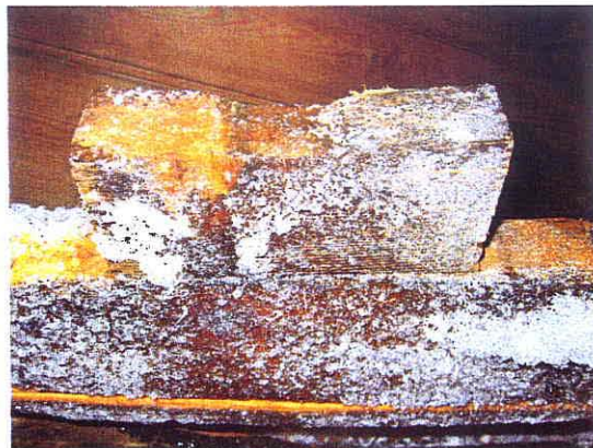
TIMBER SPACER BLOCK FROM BETWEEN COLLAR TIES AT INTERSECTIONS
