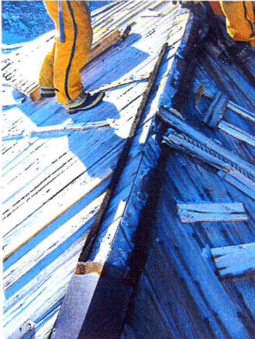
FOAM STRIPS IN PLACE FOR CAPPING TO BE FIXED OVER
