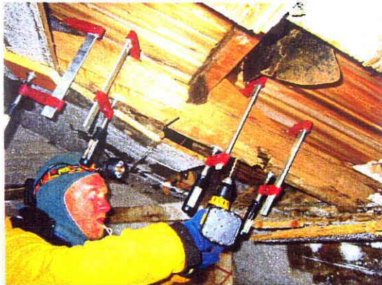
TEK SCREWS USED TO STRENGTHEN BROKEN SECTIONS OF RAFTER
