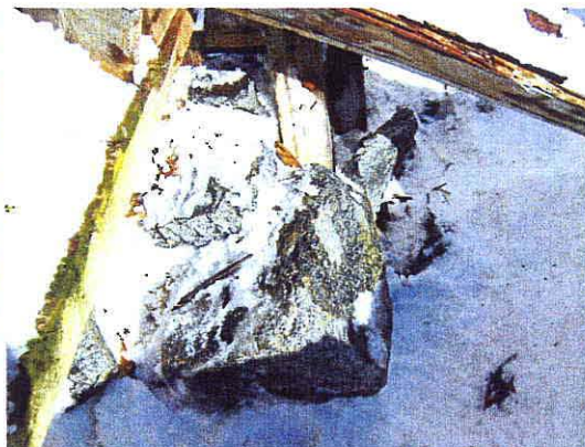
ROCKS EMBEDDED IN ICE AT BASE OF FOOTING
