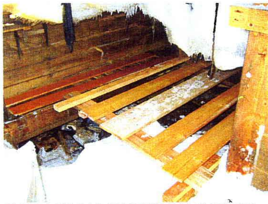
PLATFORM FOR PROTECTIVE SHEET TO BE LAID OVER READY FOR ICE EXCAVATION
