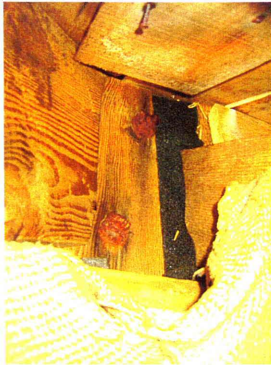
SEALING FOAM IN PLACE ON SOUTH WEST CORNER
