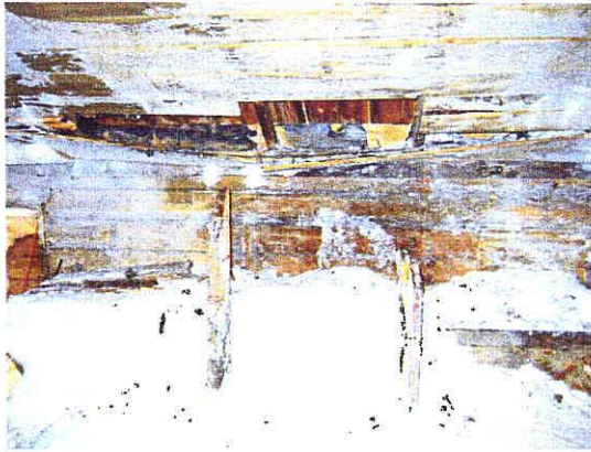
REMANANT ENDS OF COLLAR TIES PROJECTING FROM ICE MASS BELOW ORIGINAL FIXING LOCATIONS
