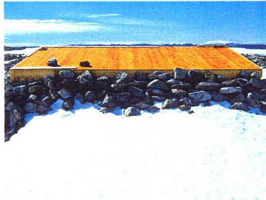
NEW COVER BOARD TO UNDER SIDE OF ROOF EAVE – NOTE LIGHT SECTION IS EXISTING SECTION
