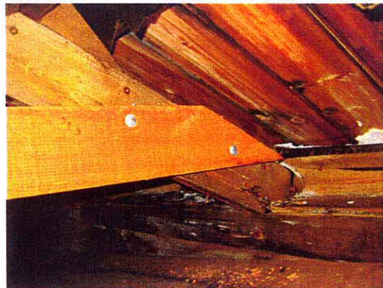
FIXING OF NEW TIE TO RAFTER
