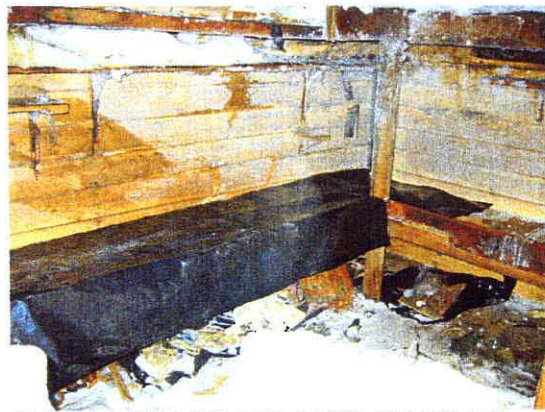
PLASTIC SHEET LEFT OVER BUNKS TO PROTECT COLLECTION OF ARTEFACTS UNDER
