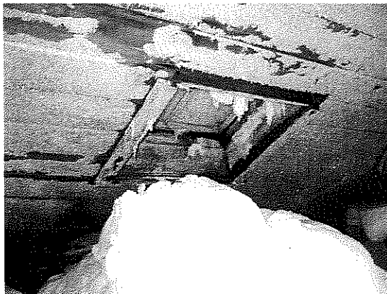
ACCUMMULATION BELOW EAST SKYLIGHT
