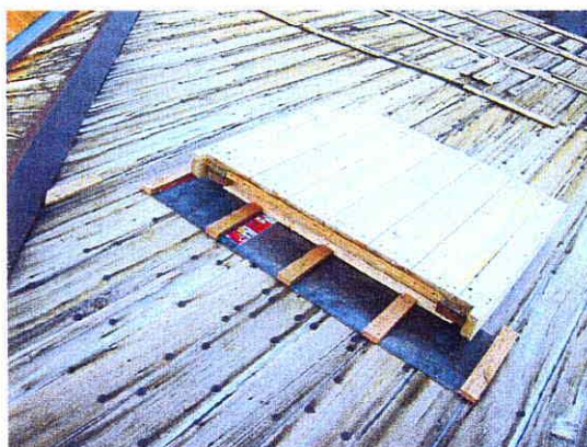
OVER BATTENS AND REMNANT CANVAS REPLACED AND REFIXED TO SOUTH SKYLIGHT
