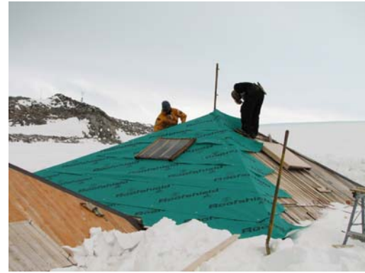
Roofshield® applied to under battens
