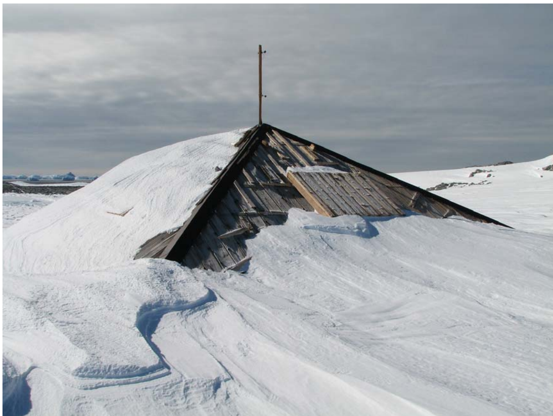
The roof of the Living Quarters as first observed by the team on their arrival at Cape Denison, October 2006
