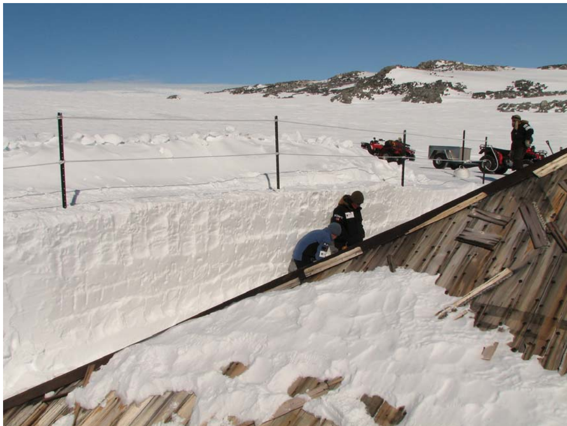
Safety fence on the southern side of the Main Hut
