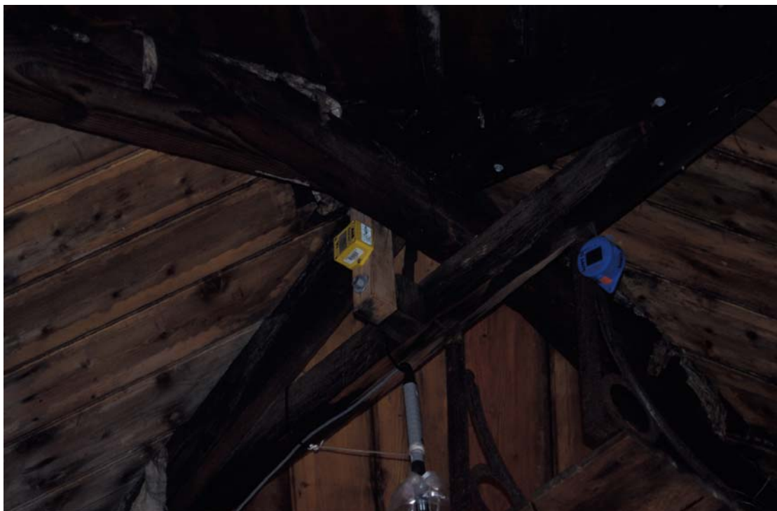
Vibration, Vaisala and Tinyview data loggers at the apex of the living quarters
