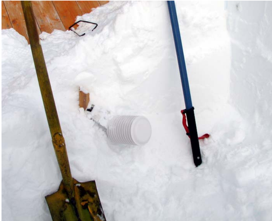
Damaged sensor housing located above the Workshop door
