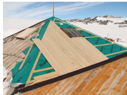
Over cladding with Baltic pine tongue and groove timbers
