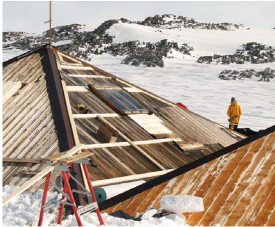
Under battens – north roof plane
