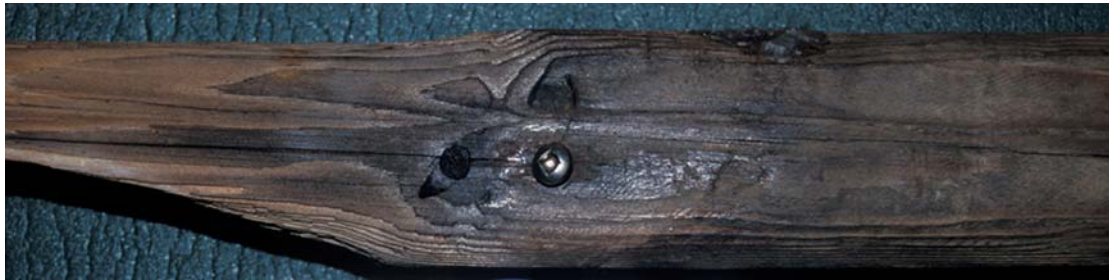
NE face of the flagpole showing historic and modern fastenings (tack and screw respectively) used to attach flashing at the apex
