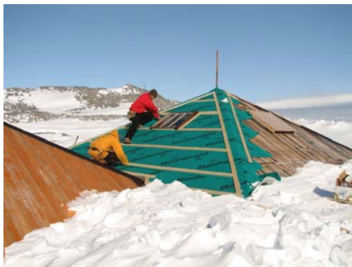
Battens attached to Roofshield® membrane
