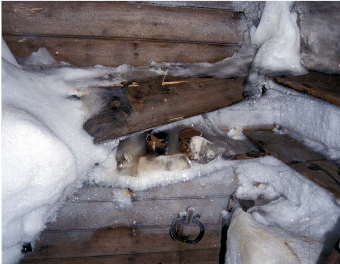
Damaged and sloping shelving in the south east corner of the Workshop
