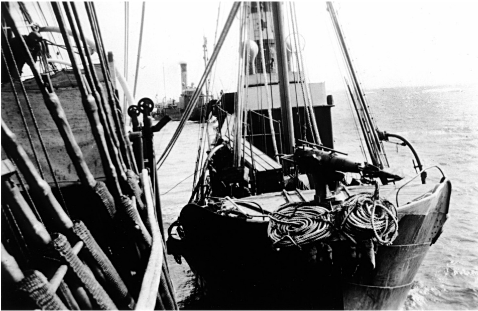
Plate 23. Harpoon gun on the bow of a whale chaser (BANZARE, Photo: T. H. Johnston)
