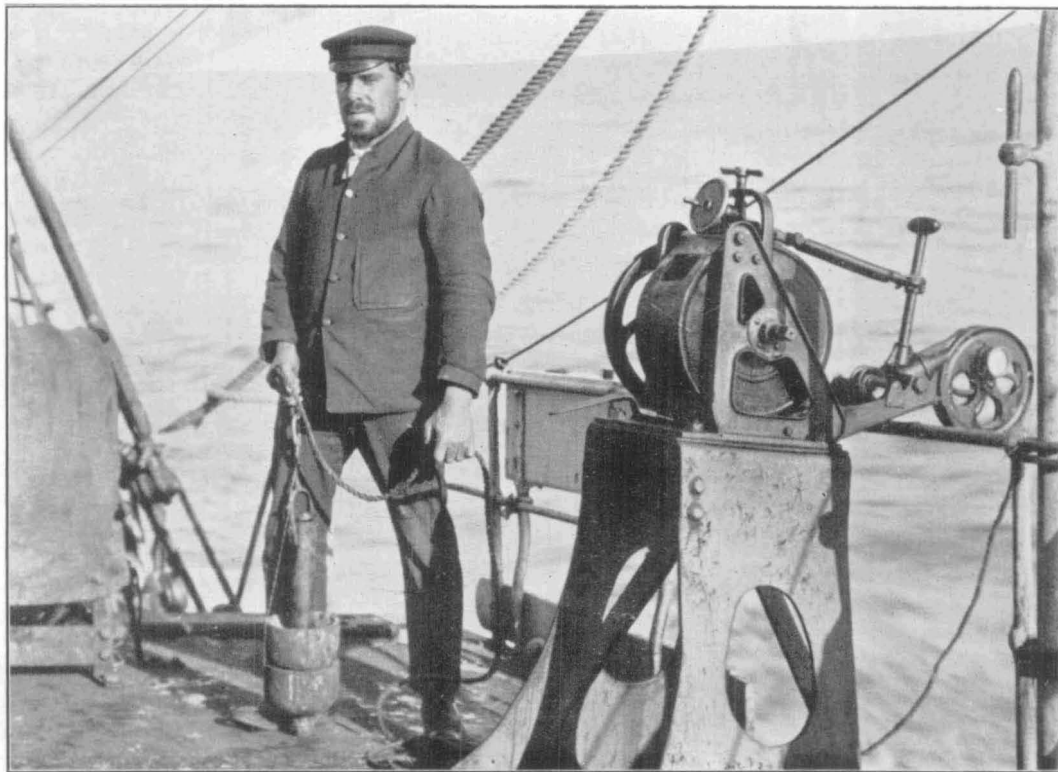
FIG. 2.—SHOWING THE BAILEE DRIVER WITH WEIGHTS ATTACHED READY FOR SOUNDING.
