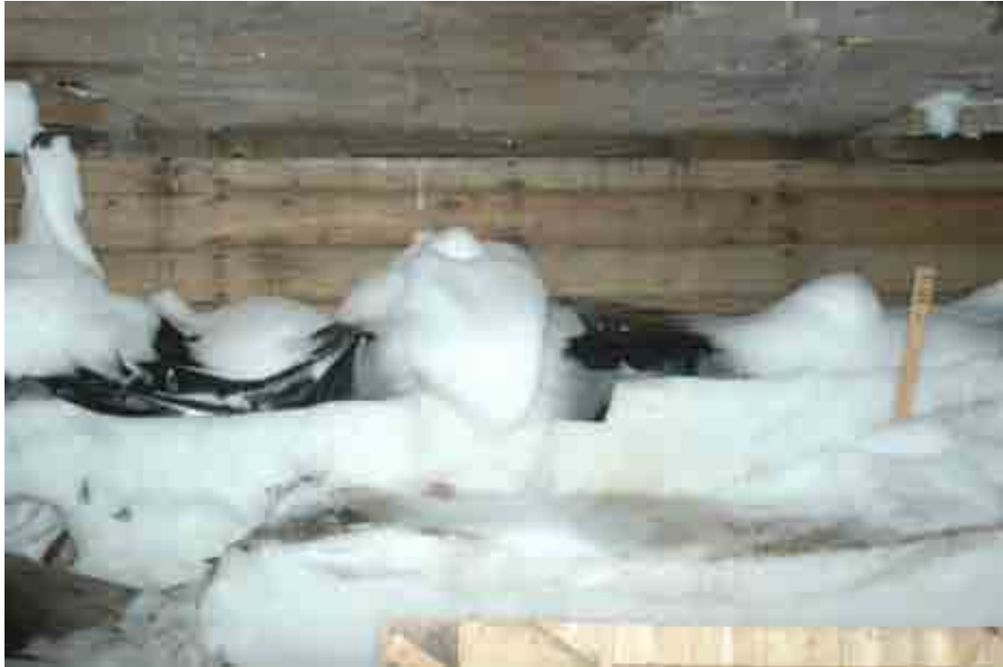
Fresh snow ingress on the internal north wall of the workshop
