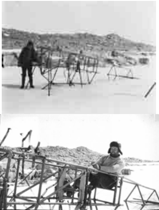
Figure 10: from BANZARE 1931: indication of the amount of metal in the airframe. Pilot Eric Douglas is seen sitting in the frame in the right hand picture, on the left an unknown man (possibly Frank Hurley) gives scale to the frame. (Photo Sally Douglas collection)
