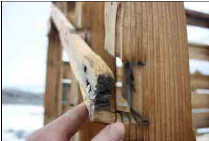
An example of one of the braces on Transit Hut with a sheared screw
