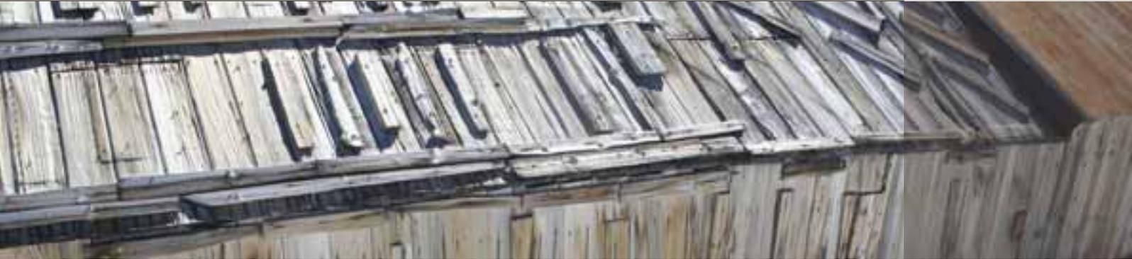
The walls and roof, both inside and outside, were of tongued and grooved pine-boards, made extra wind-proof by two courses of tarred paper. As rain was not expected, this roofing was sufficient. There were four windows in the roof, one on each side of the pyramid. We should thereby get light even though almost buried in snow.
